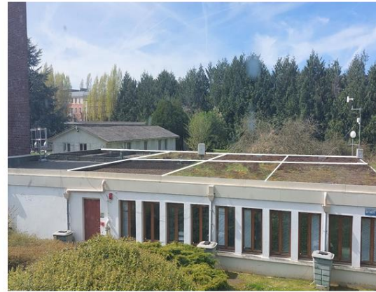
Horizontal view of the green roof (Trappes)
