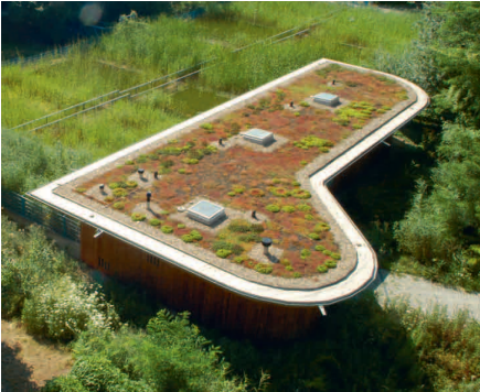
Image left: View of a soil filter for rainwater evaporation and a visitor centre (with green roof), housing a multistage greywater recycling facility (close to Potsdamer Platz, Berlin)
