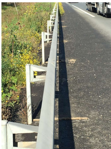
Figure 91 : Galvanized steel safety barrier separating the biofiltration swale from the road surface
