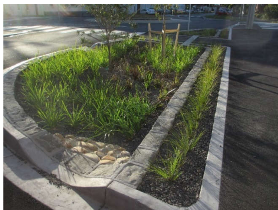
Figure 6 : Stormwater biofilter (Payne, 2017)
