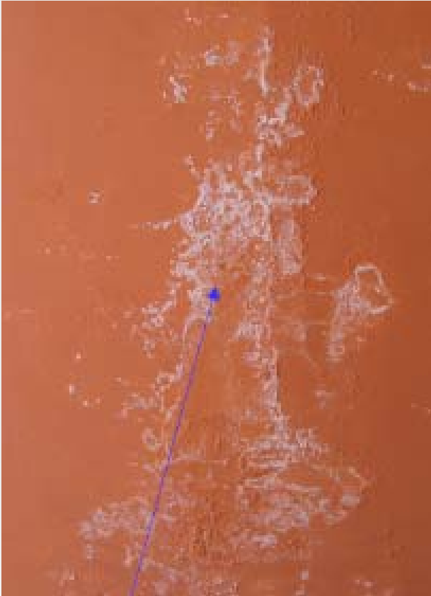
Formation of efflorescence and Formation of bubbles
